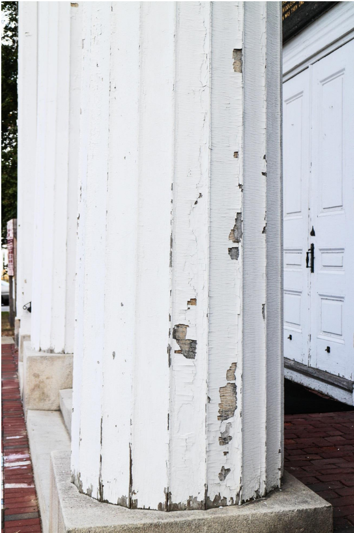
Columns on the front portico show serious signs of wear.
